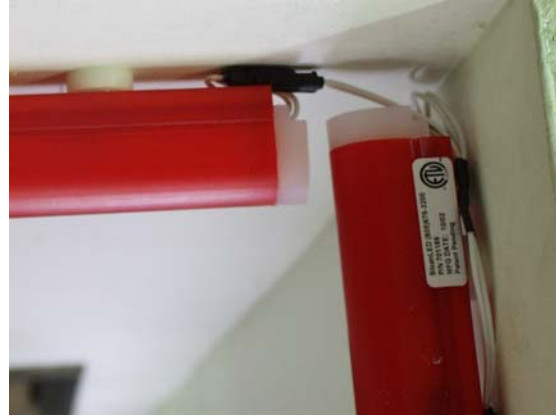
Inside corner detail showing a \frac{1}{4} " gap for expansion. Figure 20
