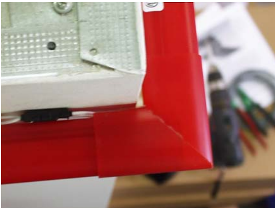
Outside corner detail showing the corner joint cover snapped in place. Figure 21
