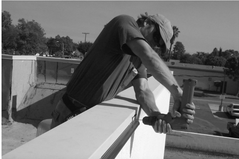
Drilling mounting button holes for an LEDStripe section Figure 4
