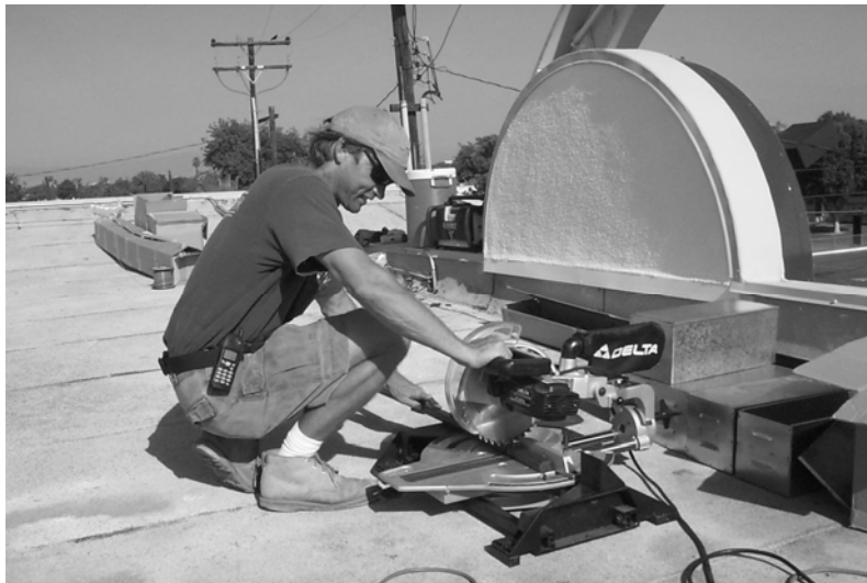
Cutting a LEDStripe section to length to fit the end of the building Figure 14
