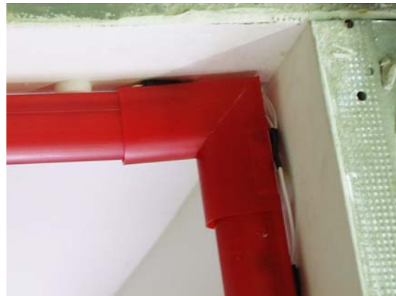
Inside corner detail showing the corner joint cover snapped in place. Figure 22
