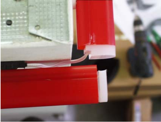
Outside corner detail showing a \frac{1}{4} " gap for expansion. Figure 19
