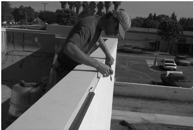
Figure 3. Marking the mounting button location
